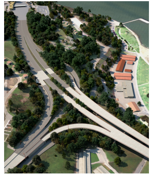
Aerial view of Presidio Parkway. Courtesy of Parsons Brinckerhoff.
